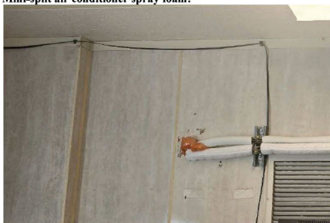
Mini-split air conditioner spray foam:
