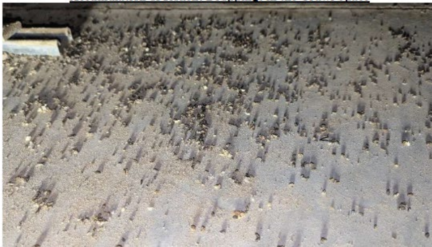
Accumulation of Rodent Droppings in the Crawl Space
