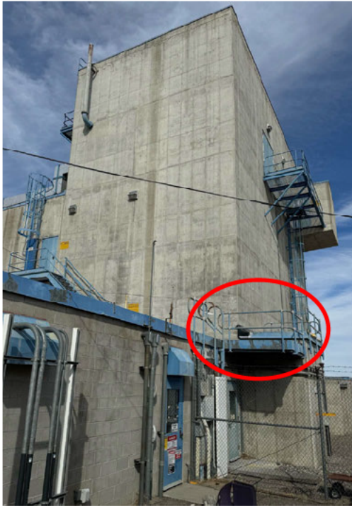
Picture 1-Location on 242S Evaporator Roof
