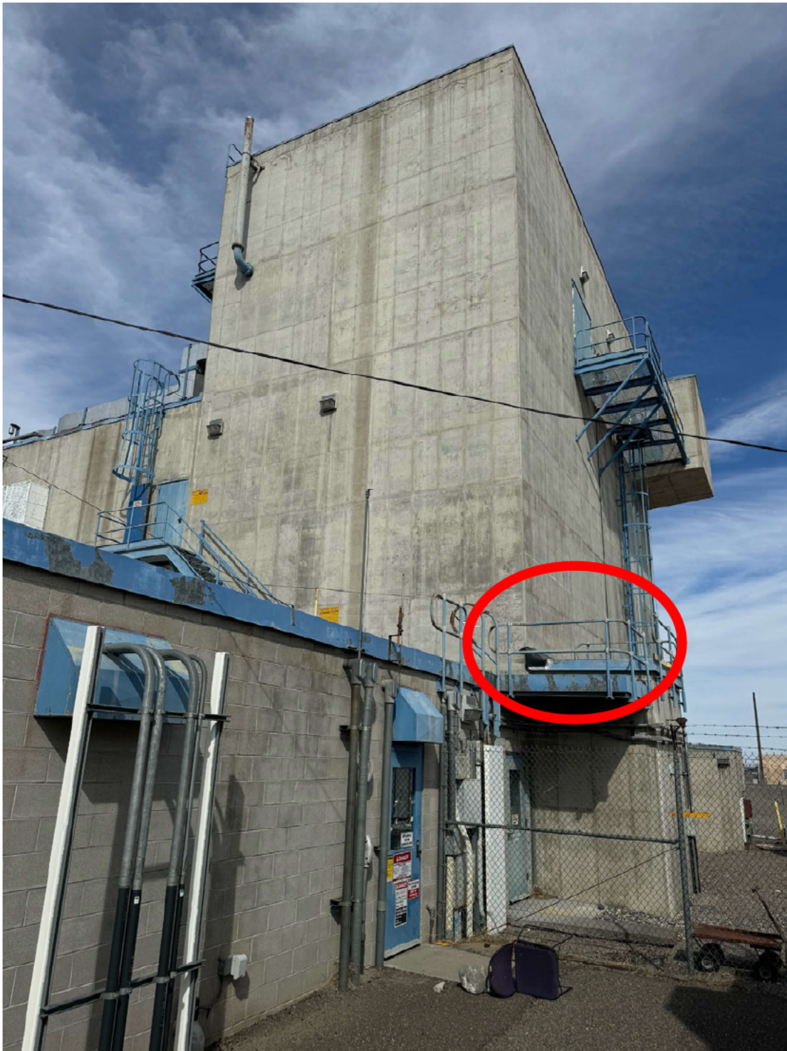
Figure 1. 242S Evaporator south side roof where odor event occurred.
