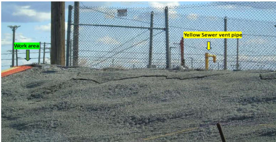
Picture 1: the yellow sewer vent pipe and location the workers were.
