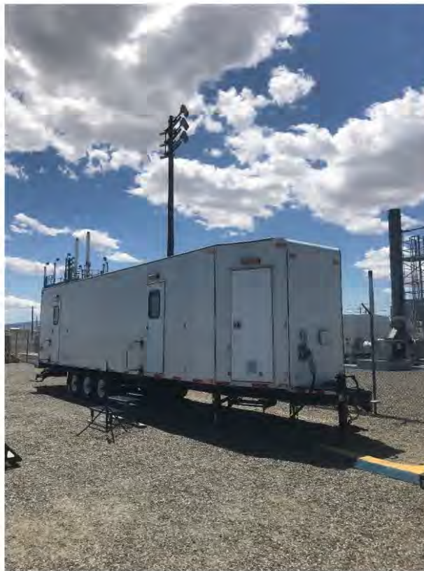
Figure 2-14. Trailer Located Along the East Fence Line of AP Farm.
