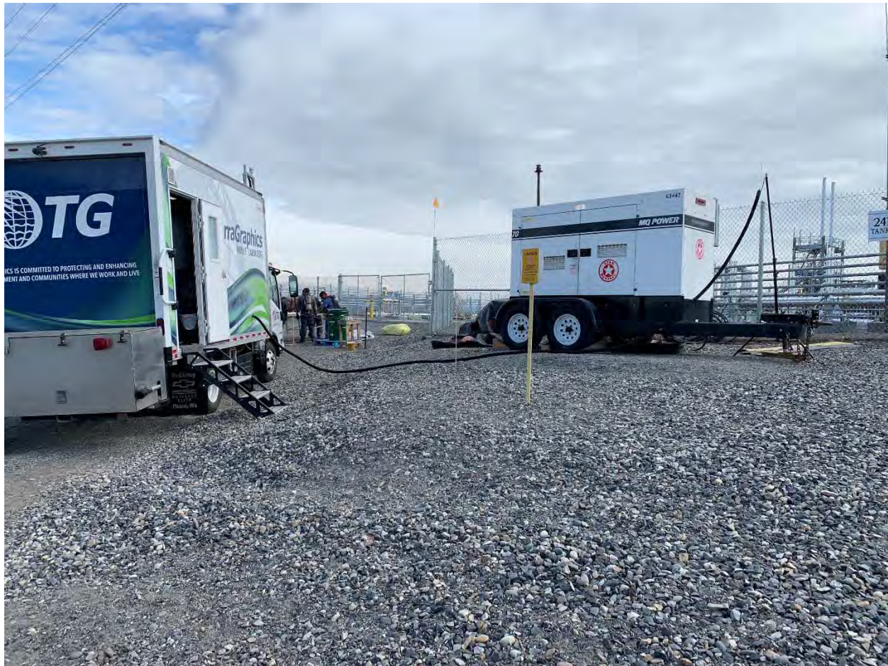
Figure 5-2. Mobile Laboratory Monitoring of Generator #1.
