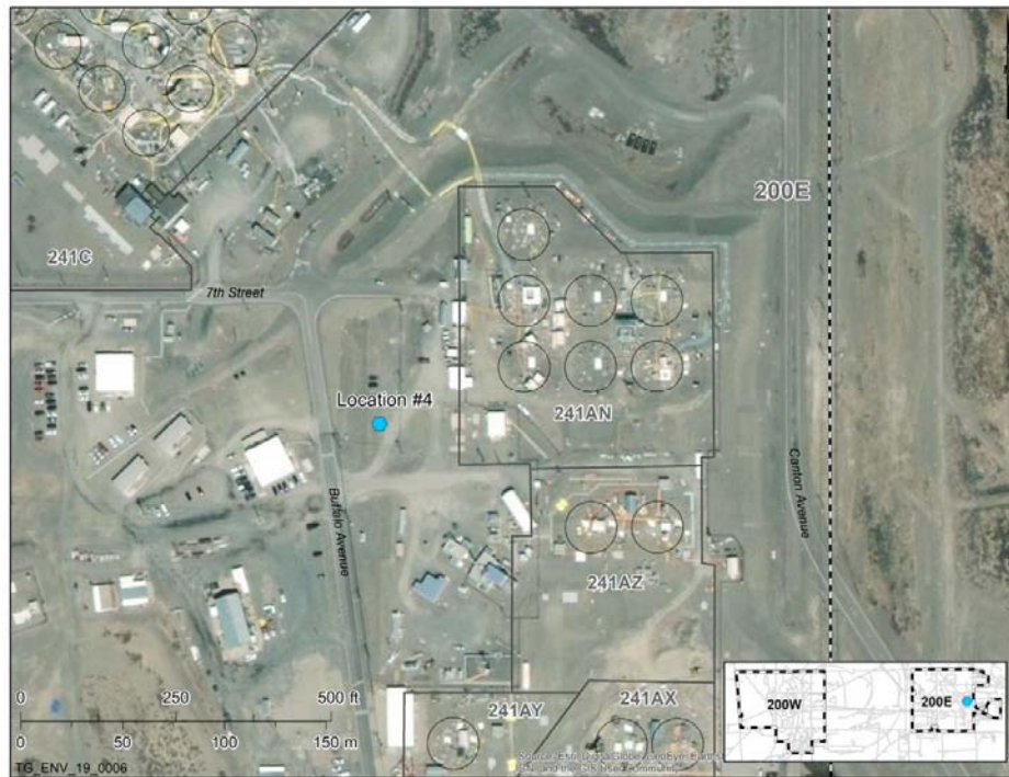
Figure 2-1. Mobile Laboratory Site #4 for the Duration of the Monitoring Period.
