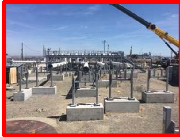
Figures 2. (Right) Installation of Weldments (Photo courtesy of Mark Allen)
