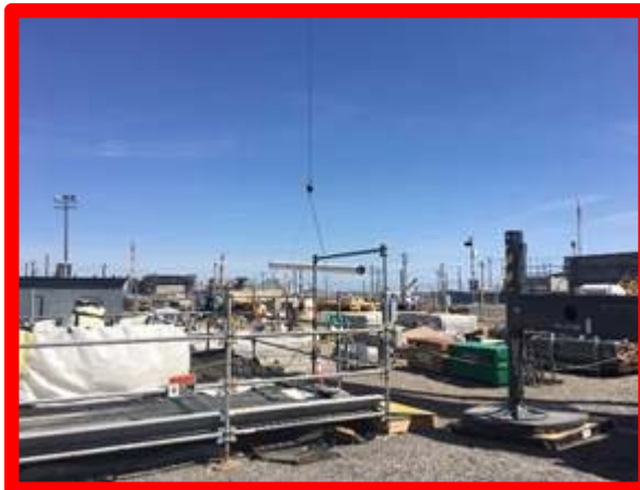
Figure 1. (Above) Installation of Weldments (Photo courtesy of Mark Allen)
