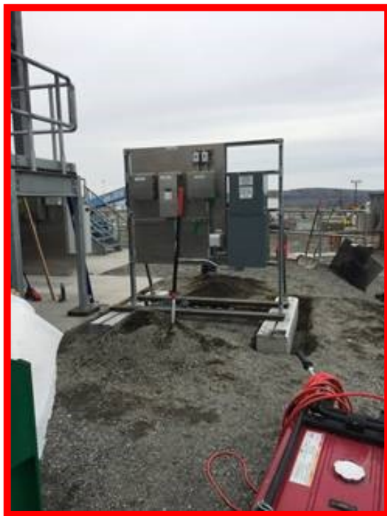
Figure 1. (Left) A-Farm Exhauster Electrical Rack Installation (Photo courtesy of Mark Allen)
