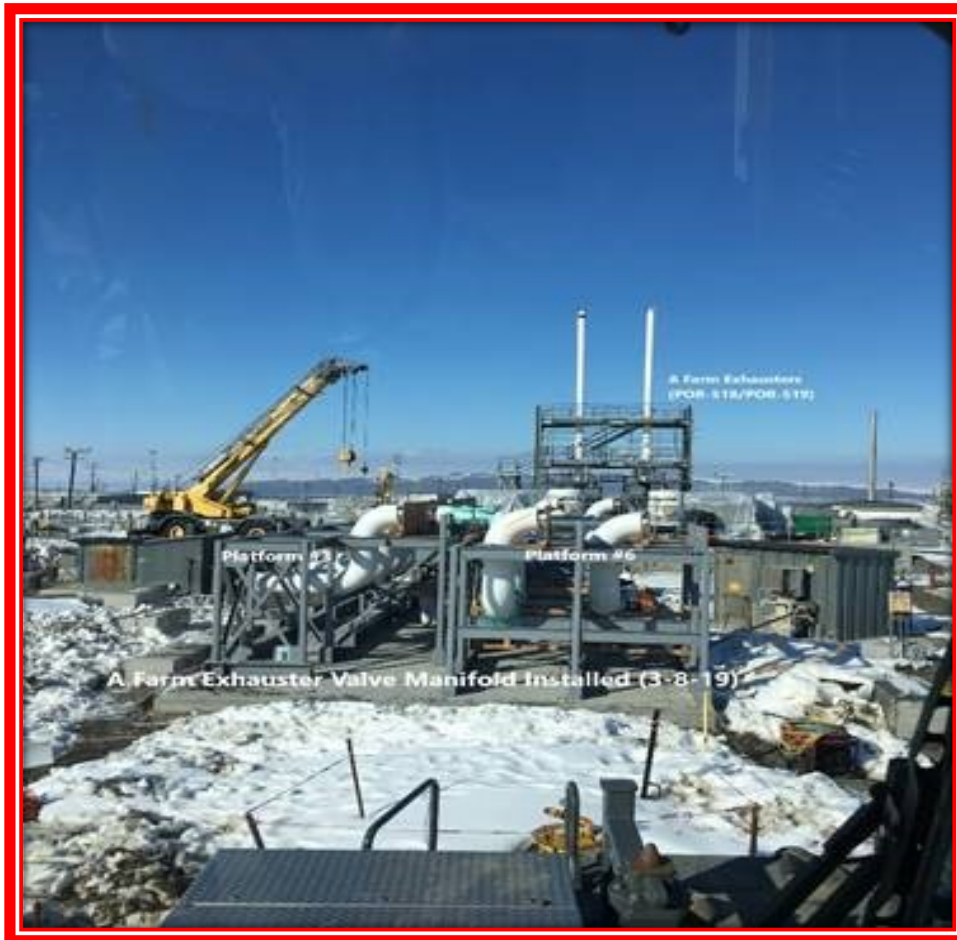
Figure 4. (Left) A Farm Exhauster Valve Sub- assemblies. (Photo courtesy of M. Allen.)
