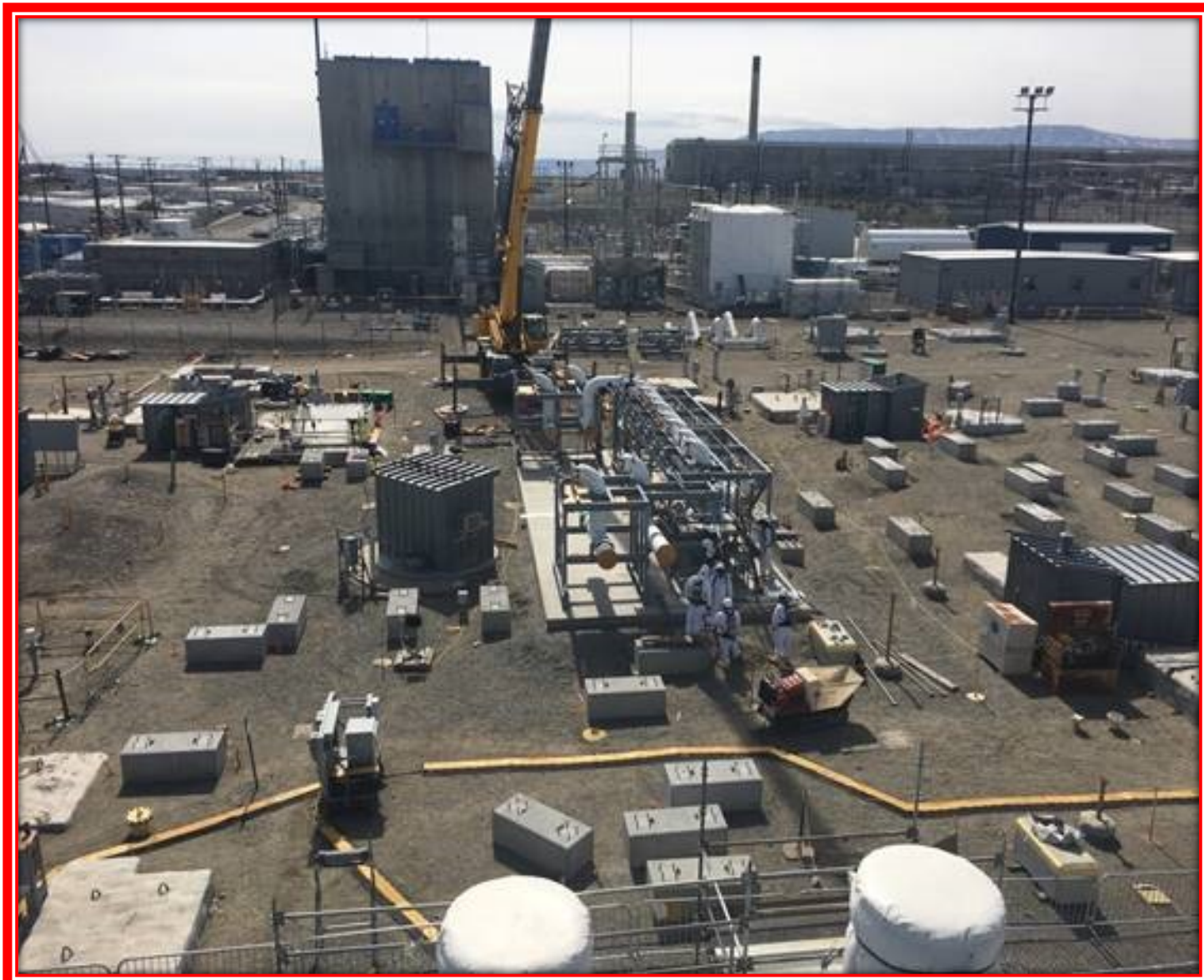
Figure 5. Ventilation Ducting Support- Block Installation (Photo courtesy of M. Allen.)
