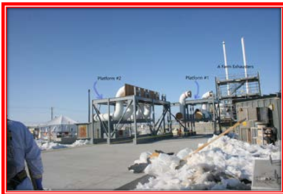
Figure 1. A Farm Exhauster Valve Manifold Construction – 2 of 6 Subassembly Platforms Installed.
