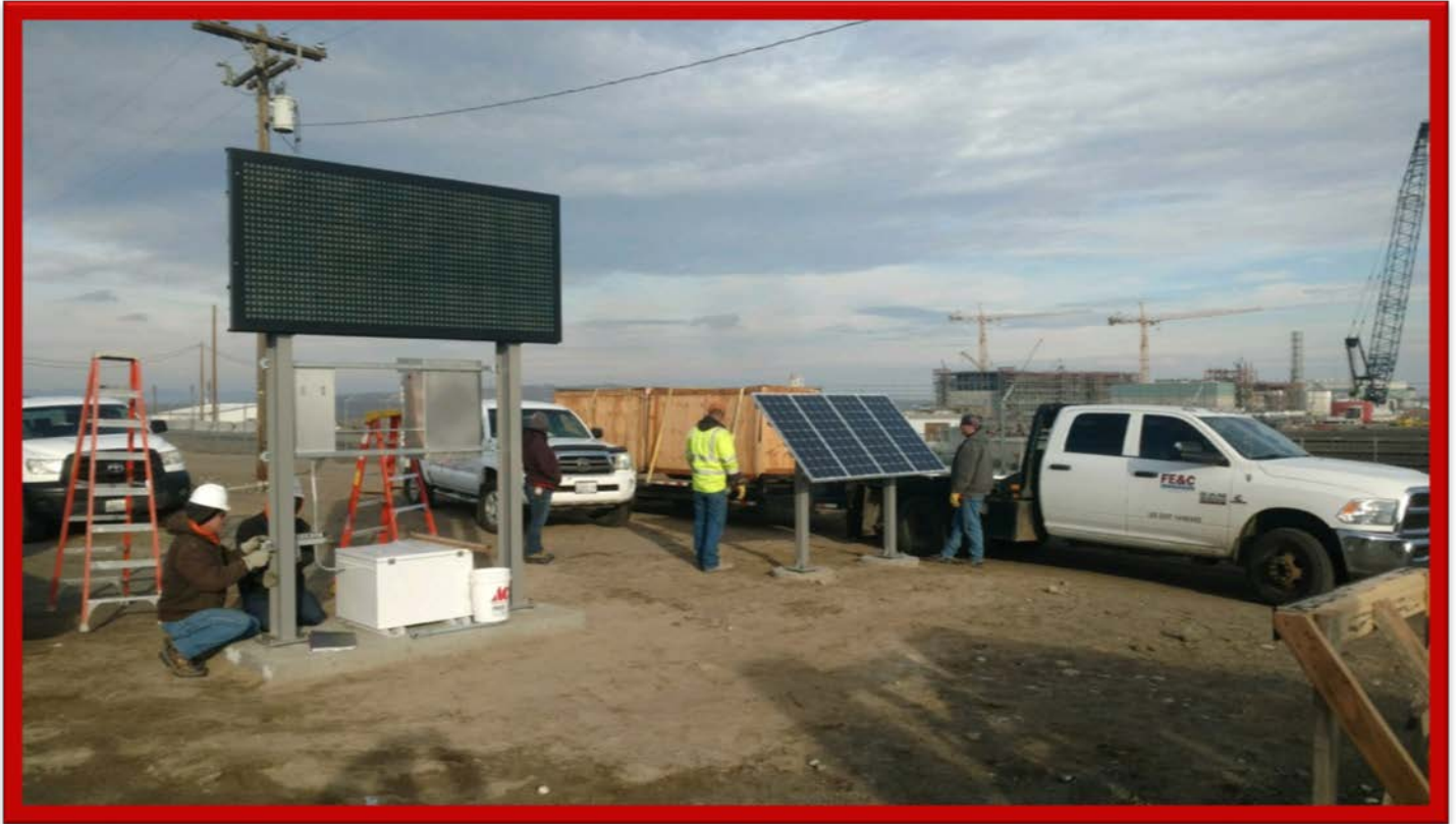
Figure 8. Reader Board and Solar Panel Installation – December 2018 (Photo courtesy of Bobby Nelson.)
