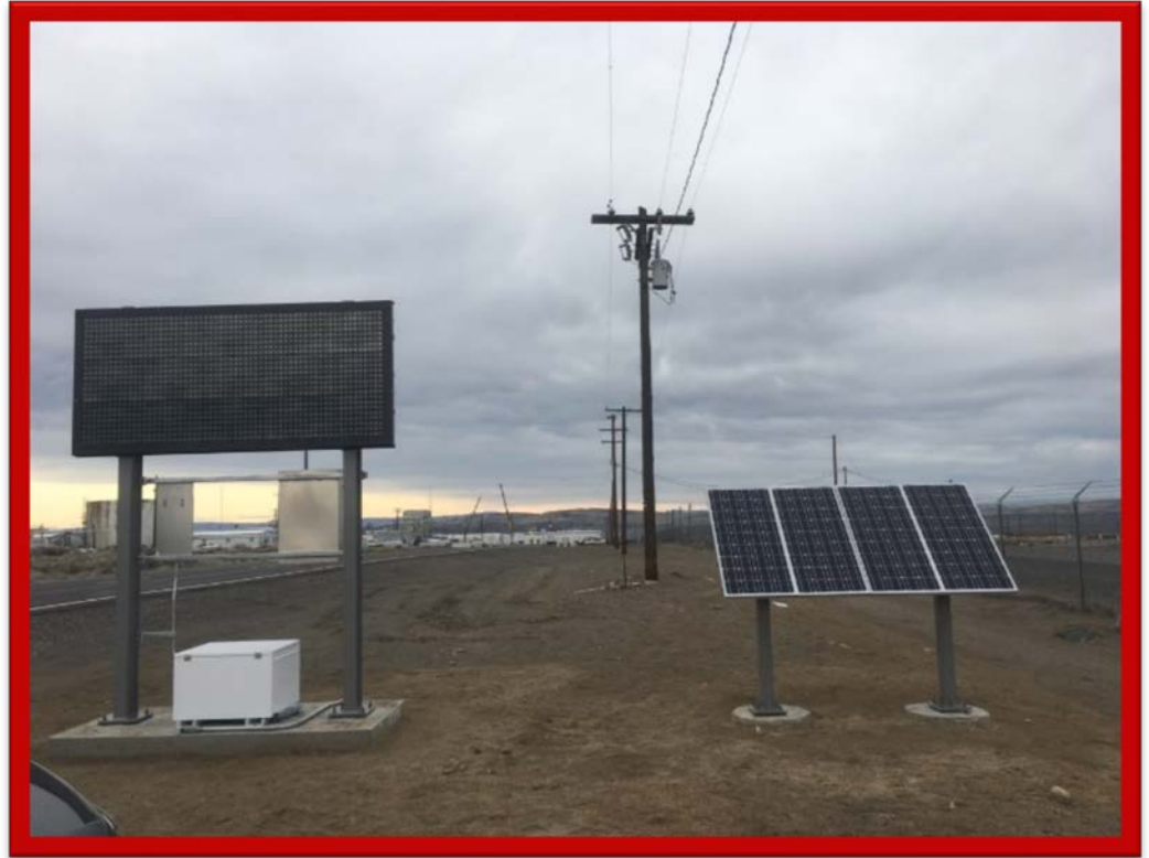
Figure 9. (Right) Reader Board and Solar Panel Installation Complete – December 2018 (Photo courtesy of Bobby Nelson.)
