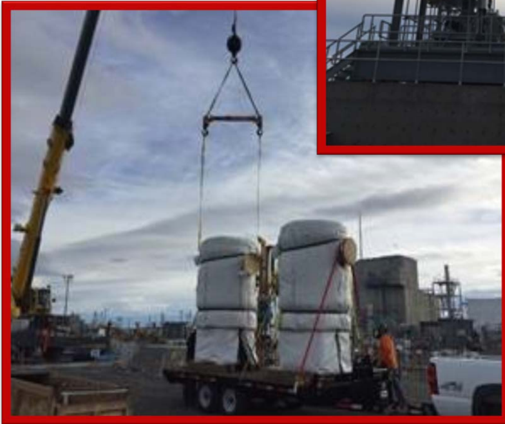
Figure 7. A Farm Exhauster Moisture Separator Installation (Photo courtesy of M. Allen.)
