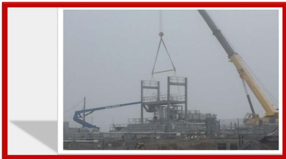
Figure 5. A Farm Exhauster Installation Activities continue in November 2018 (Photo courtesy of M. Allen.)
