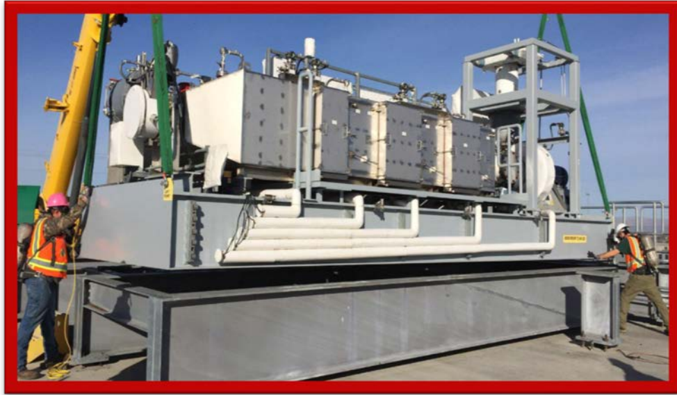
Figure 4. A Farm Exhauster Stacks – Preparations for Installation in October 2018 (Photo courtesy of M.Allen.)
