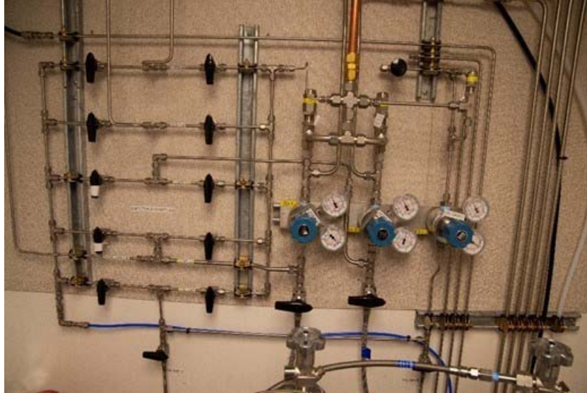
Figure B.10. Inside the trailer north end East end valve manifold (COPC#1, 3 &4).
