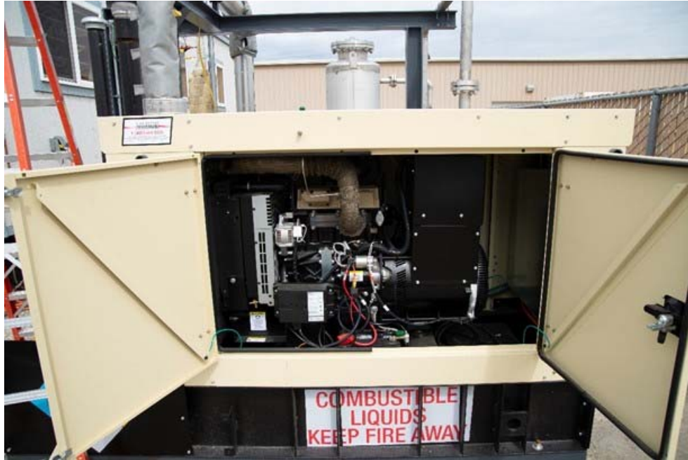
Figure A.6. The Kohler KDI1903ESM Diesel Engine Spec 6D08E1-1 (S/N 4728402750) rated at 28 BHP at 1800 rpm with Decision-Maker 3000 controls. Engine power 19-37KW with 1.861 liters displacement. (Engine family HKHXL2.49ESM.) On the lower right image is the connected Kohler 15REOZK 15 kVA Generator (S/N SGM32LMWJ).
