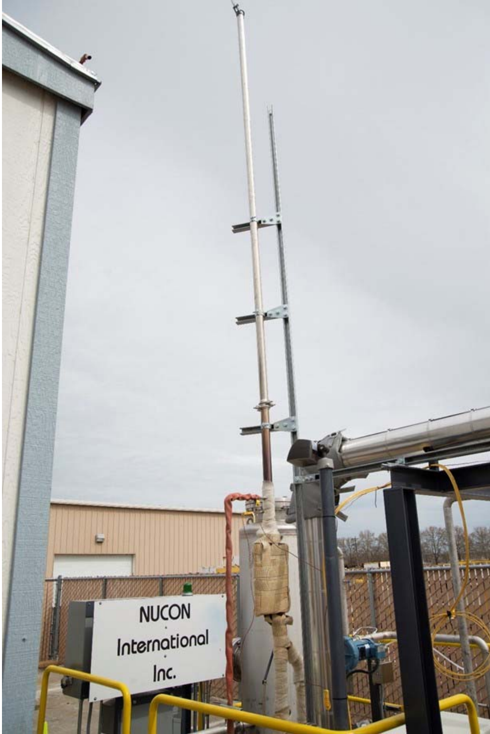
Figure A.8. Exhaust gases then exit the 2-in. exhaust muffler and then out the extended a 10-ft-long 2-in. exhaust pipe that was added to the muffler
