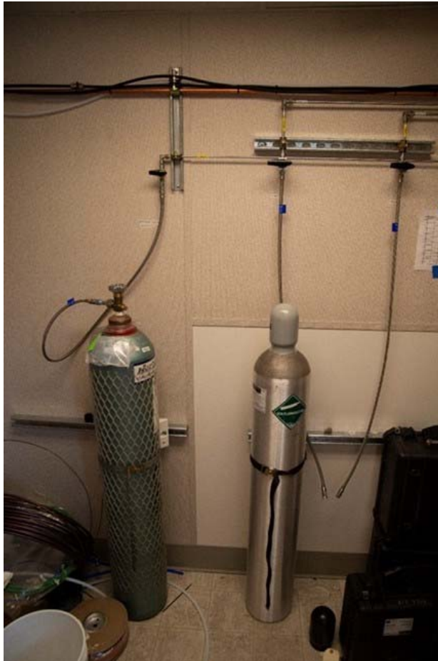
Figure B.11. Inside the trailer north end bottle rack and valves (COPC#1, 3 &4).
