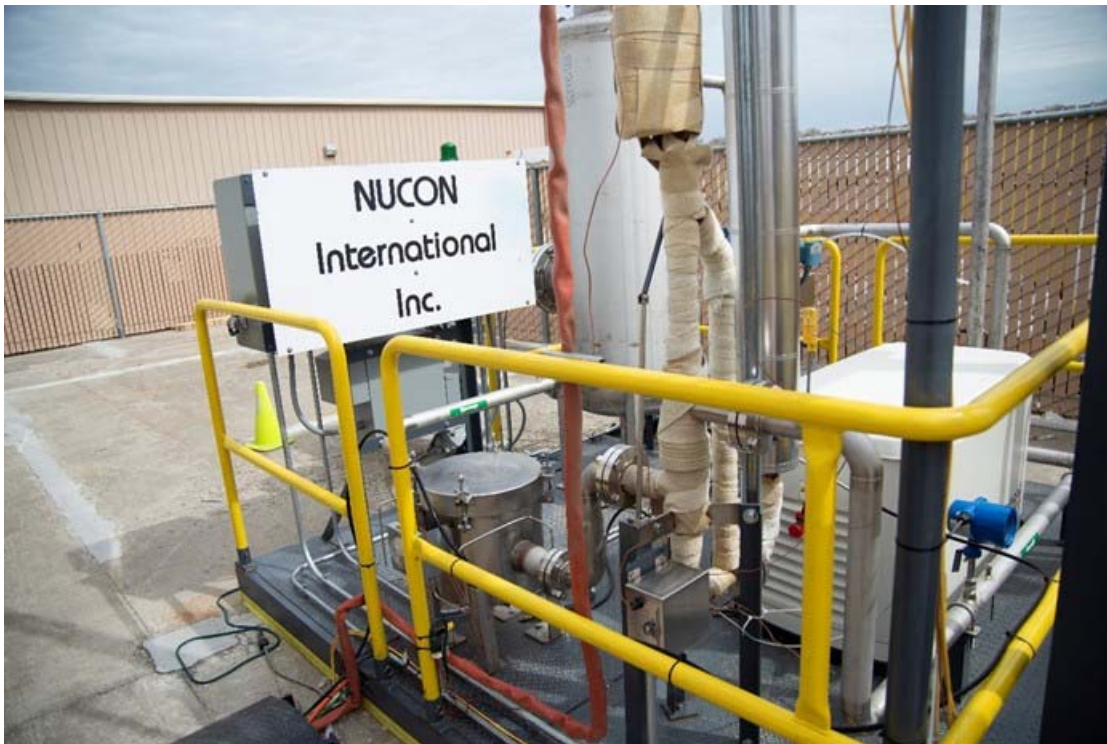
Figure A.4. (Looking northeast) Under the white and tan insulation fiberglass wrap is the ambient air inlet to the heat exchanger that used exhaust air to heat the ambient air before going into the MERSOB ® filter. This is followed by the Yellow K type Thermocouple TT-103 outlet air temperature after the heat exchanger and the second particulate HEPA filter housing.
