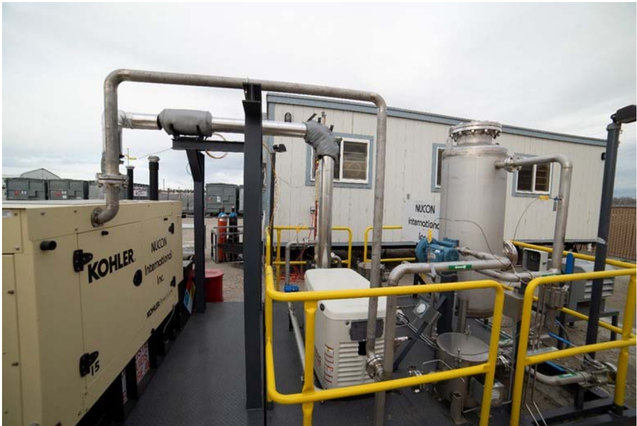
Figure A.3. (Looking west) Inlet air pipe wrap around the skid. A Fox Thermal Instruments, Inc. Model FT1-06IDDP1 serial # F00780 Flow Meter set to 0 to 60 scfm per vendor-approved change. (FT-101). Then the Yellow K type Thermocouple TT-102 before the flow is warmed in the heat exchanger. The tan box houses the propane engine and generator that were disconnected for the testing.
