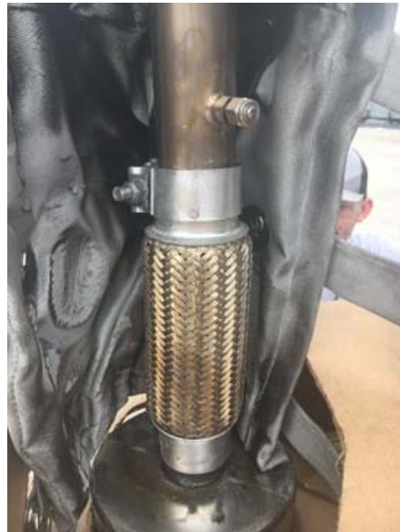
Figure A.13. The top connection to the 4SX-15REOZK Catalytic Purifier muffler emissions control device (i.e., diesel oxidation catalyst) with the insulation pulled back.
