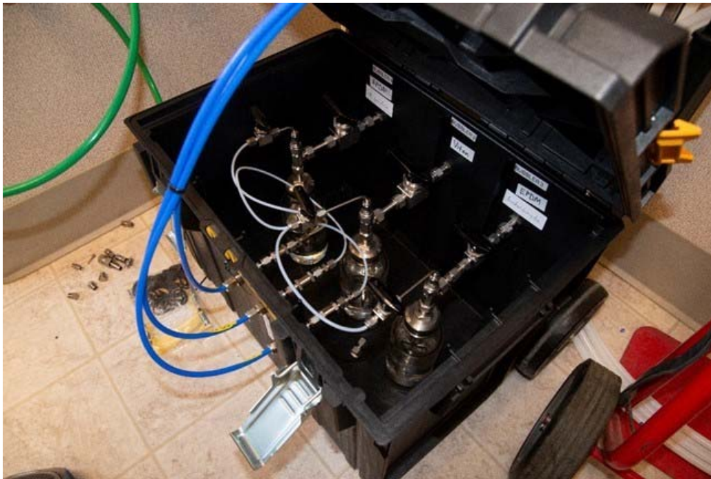
Figure B.12. The liquid bubbler system (on the Northwest wall inside the trailer).
