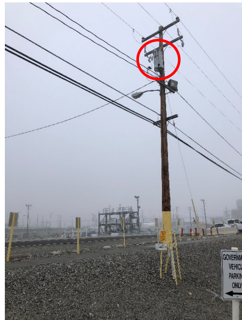
Utility Pole and Transformer C6692L
