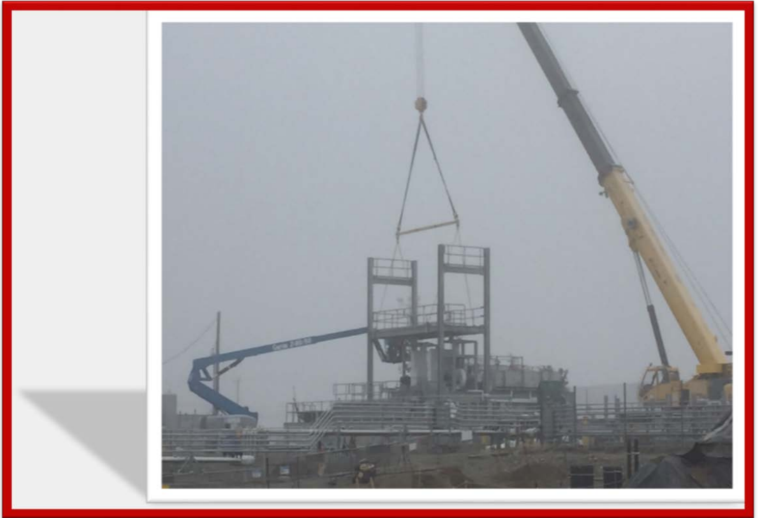
Figure 2. A Farm Exhauster Components Installation (Photo courtesy of J. Laurenz)
