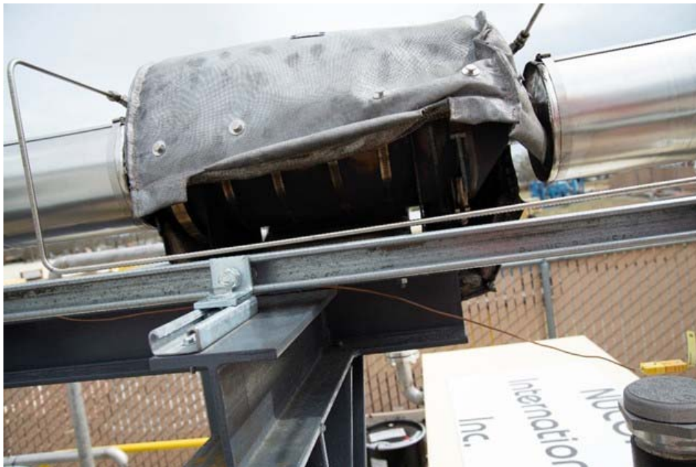
Figure A.7. Directly behind the label is the 4SX-15REOZK Catalytic Purifier muffler emissions control device (i.e., diesel oxidation catalyst) manufactured by Catalytic Exhaust Products with the second photo being the diesel particulate filter 758SXS-SC by Catalytic Exhaust Products.
