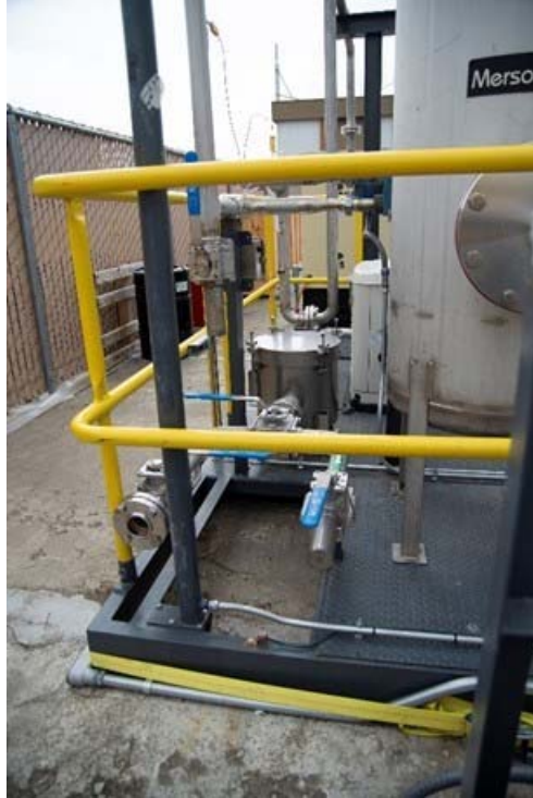
Figure A.2. (Looking south) The metal particulate screen (60 mm x 150 mm) connected to the three-way valve. This was the sole path through which ambient air was introduced to the system during steady state testing. The piping on the skid was 316/316L Stainless Steel WLD 2-in. schedule 10S. Also visible is the first particulate HEPA which is also called the demister (14-in.-diameter x 14-in.-tall outside housing dimensions) filter housing. Both HEPA filter housings have an installed Astrocel® I High Efficiency Particulate Air (HEPA) Filter flow tested for 50 cfm (size 8" x 8" x 5 7/8" part number 12A26J6P0A1, 900-895-503) with nominally 0.8 inches of water resistance. The filters are made by American Air Filter (see image of the west HEPA filter below). Note that one filter is in the HEPA filter housing on the east side of the skid and the second filter in inside the HEPA housing on the west side of the skid.
