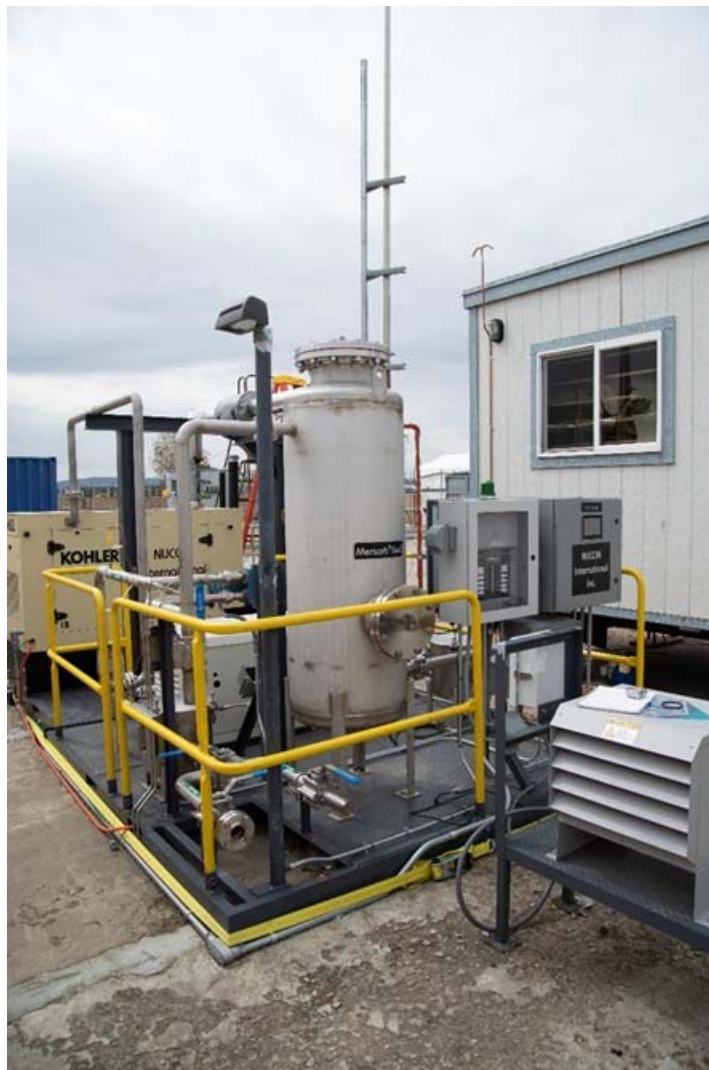
Figure A.5. (Looking southwest) MERSOB® Absorbant container made of 24-in.-diameter schedule 10S A-312/SA-312 stainless steel with a length of 64 in. NUCON had not removed the 73 kg of Mersorb® Absorbent that had been tested in Ohio for a ~45 minute test with mercury. (Inlet air was near the bottom and release air from the column came out near the top).
