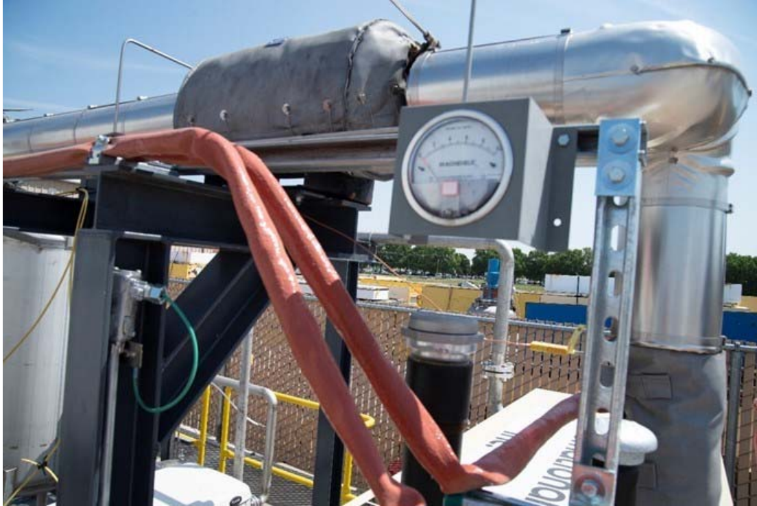
Figure B.6. Orange insulation over the heat tape on sample lines B and C can be seen going past the Magnehelic® delta pressure gauge that was added to the Diesel Particulate filter. Exhaust sample line D was also heat taped (shown below).
