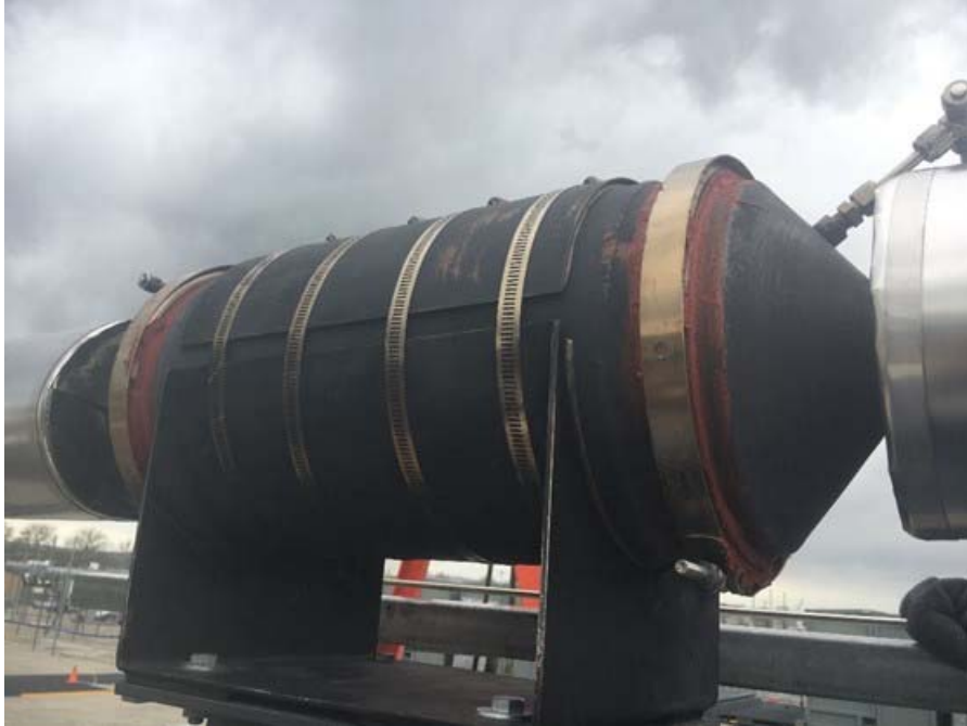
Figure A.12. The repair of the diesel particulate filter soot leak with the high-temperature seal. The insulation was removed during this pretesting repair.
