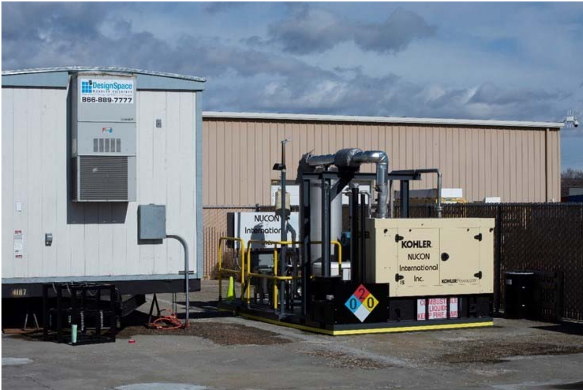
Figure A.1. The NUCON Vapor Abatement Unit (looking north) next to the Test Instrumentation Trailer. Includes the southern placed diesel skid assembly and the original northern placed propane skid.
