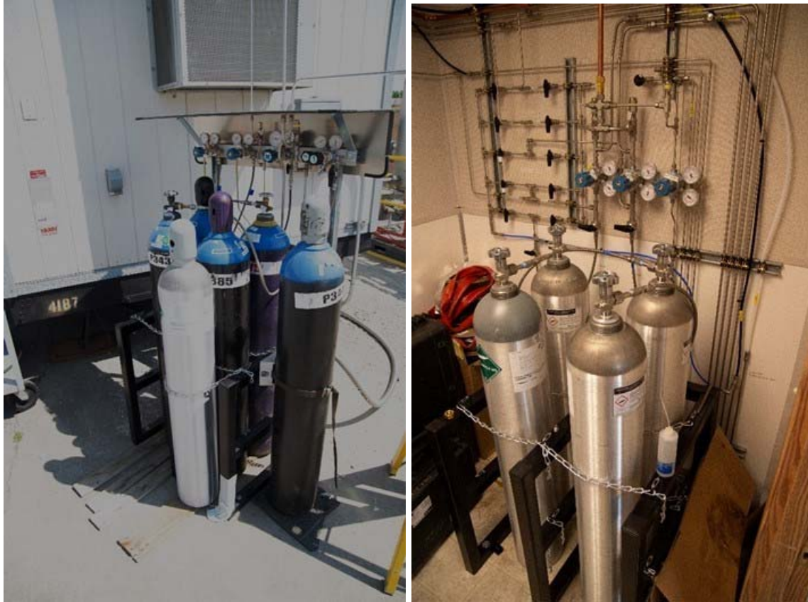
Figure B.9. Left Image - Outside bottle rack and controls (COPC # 3 & COPC #4, Ultra-Pure Nitrogen, Zero Air, Helium and other support gases). Right Image – Inside Northeast bottle rack and manifold for (COPC #1 through 4, calibration gases A and B). Below is the manifold detail.
