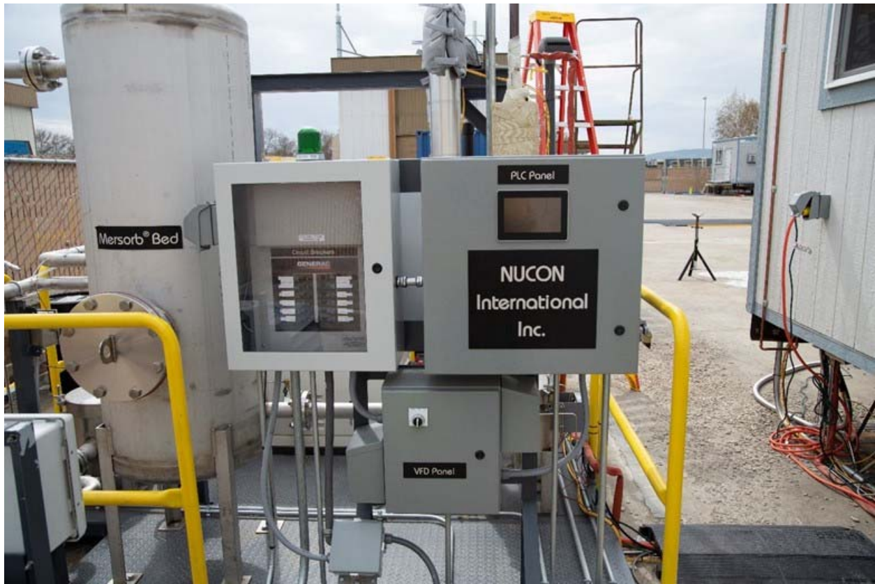
Figure A.10. Connected to the electrical output from the generator are the circuit breaker box that powers the PLC controller and the Human Machine Interface (HMI) controller and data collection.
