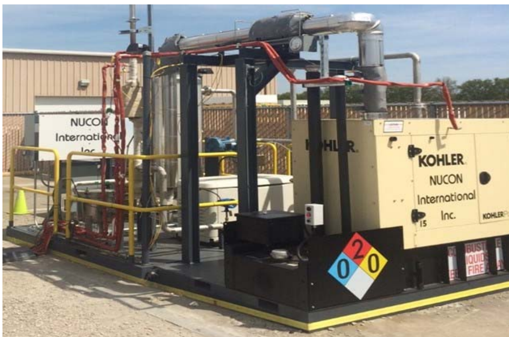
Figure S.1. Engineering-Scale Prototype of NUCON Vapor Abatement Unit
