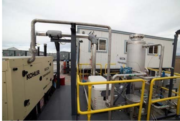
Figure 1. Photo of the NUCON VAU
