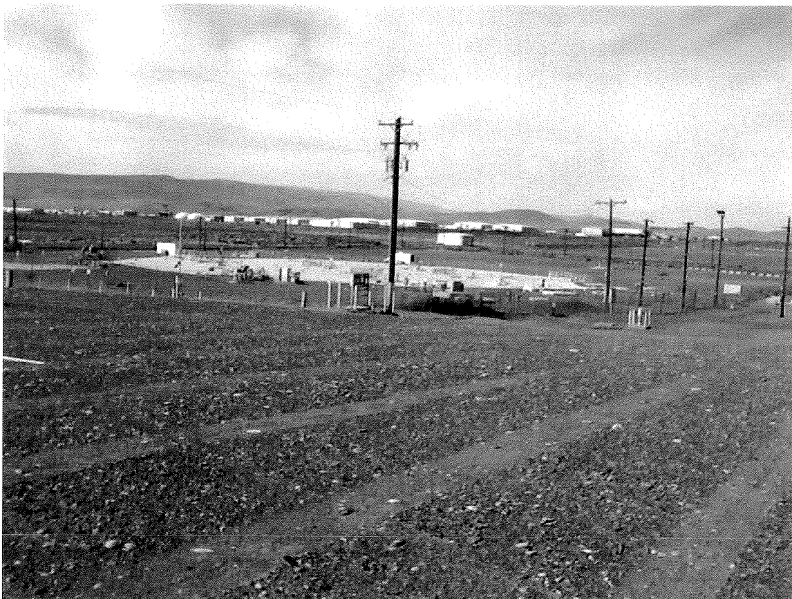
Photograph 2. Looking West toward 241-T-201 Work Area – from Location of Herbide Spraying.
