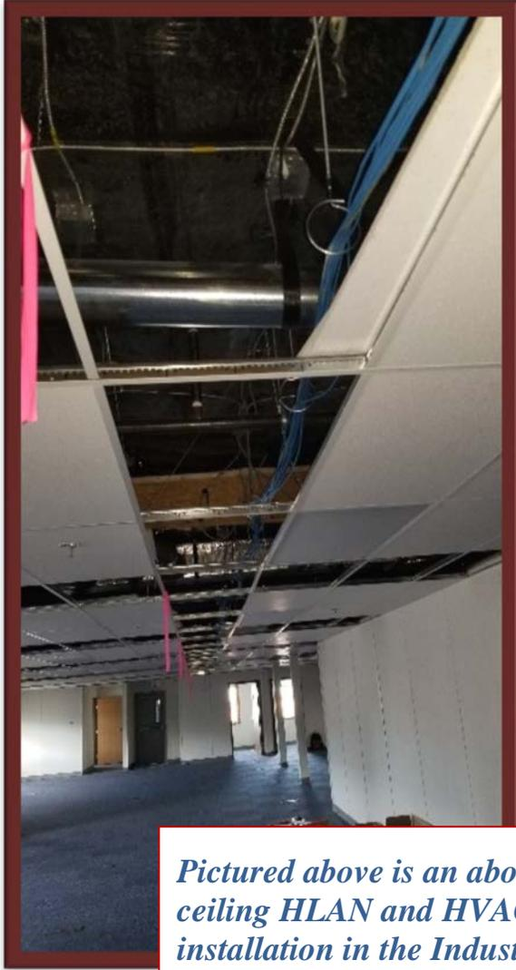
*Pictured above is an above-ceiling HLAN and HVAC installation in the Industrial Hygiene Trailer. (Photo courtesy of L. Parks-Beyer)*
