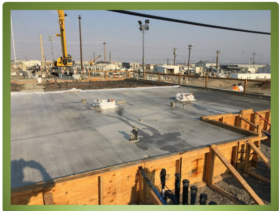
Figure 5. Completed Concrete Pour for east side of A Farm Exhauster Slab (Photo courtesy of M. Allen)
