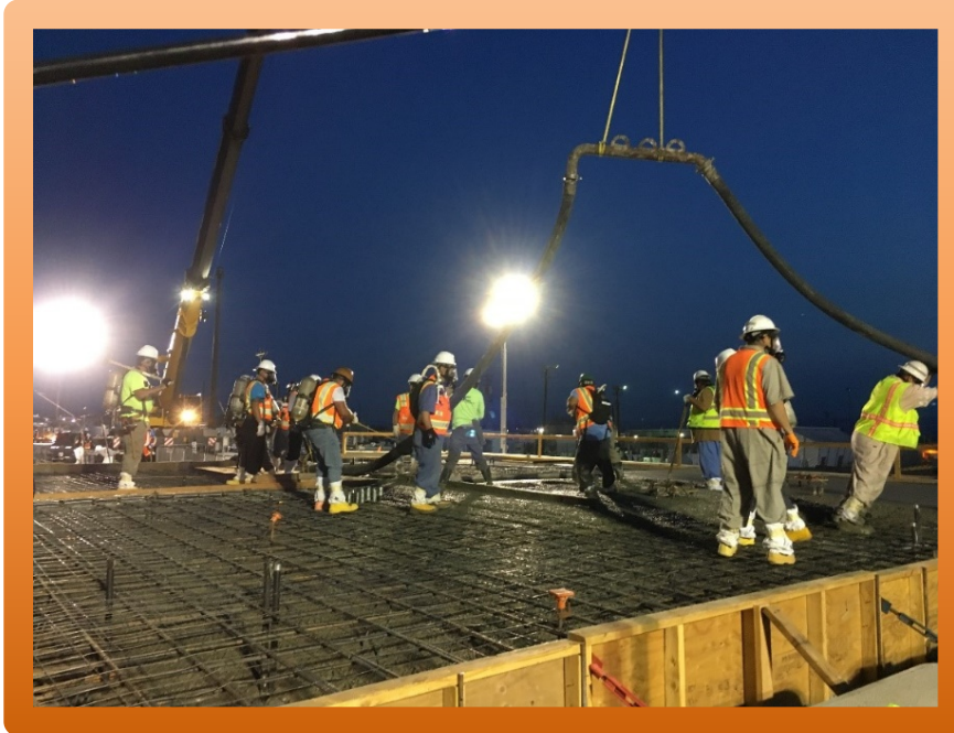
Figure 4. Installing Rebar and Pouring Concrete for A Farm Exhauster Slab. (Photo courtesy of M. Allen)
