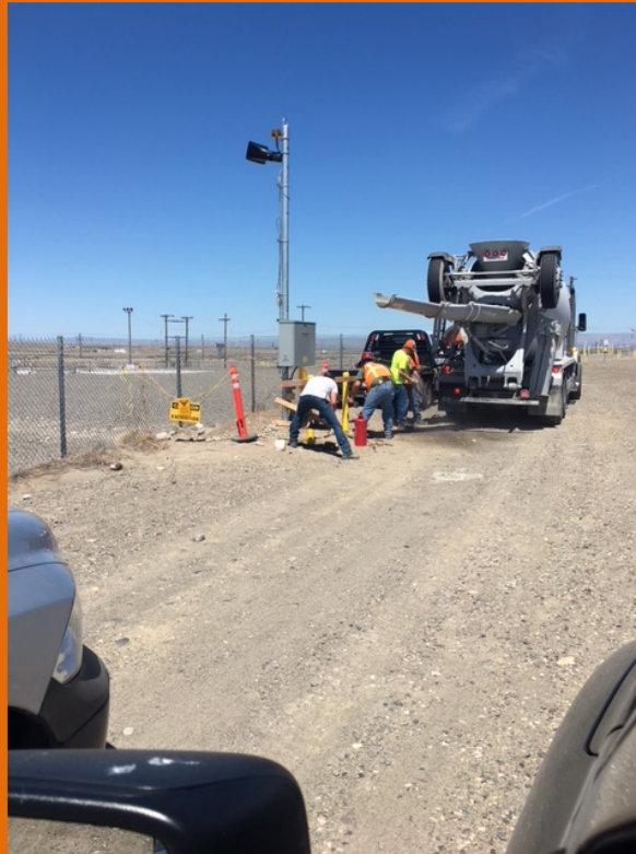
Figure 8. (Above) Backfill and Concrete Pour of Conduit Trench at B Farm Complex (courtesy of B. Nelson)
