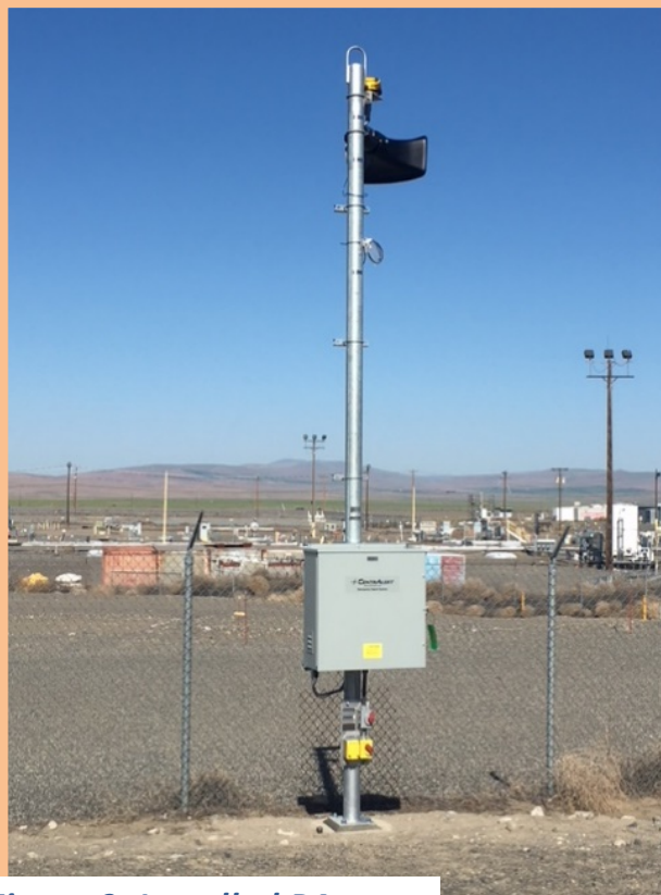
Figure 9. Installed PA System at B Farm Complex (courtesy of B. Nelson)
