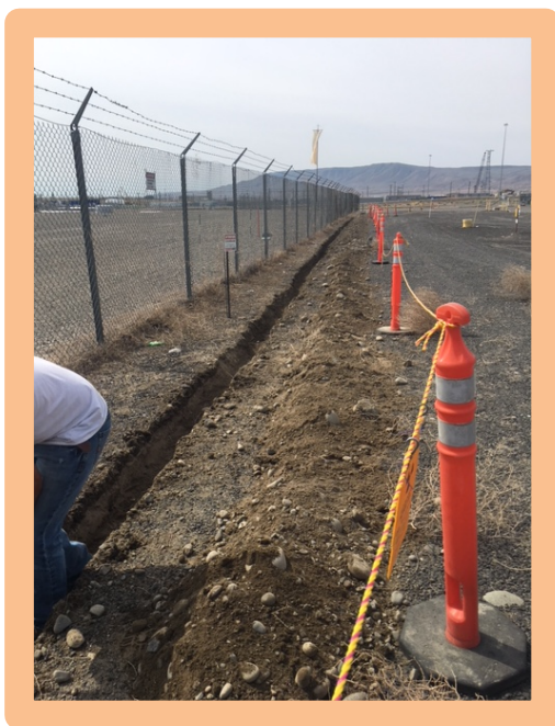
Figure 6. Trench for PA System conduit at B Farm (courtesy of B. Nelson)
