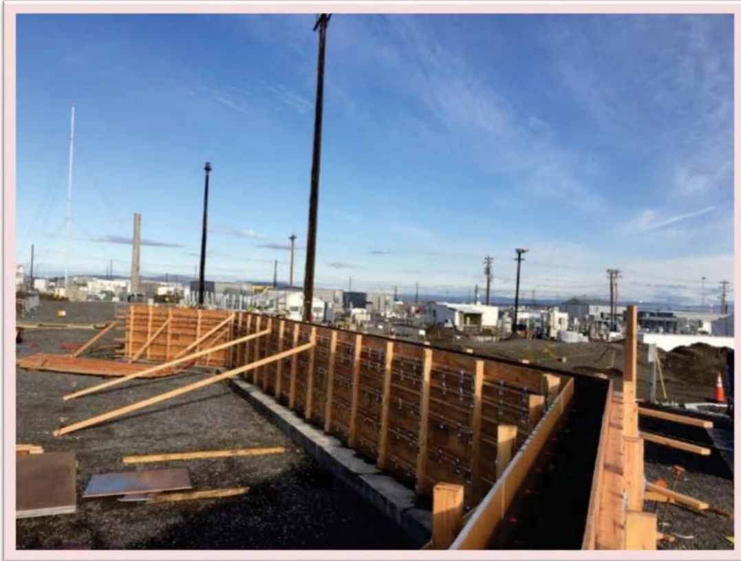
Figure 2. Pictured is an A Farm Exhauster Retaining Wall. The rebar and forms have been installed and are awaiting the concrete. For more, see KPP 4, Engineering Controls. (Photo courtesy of M. Allen.)
