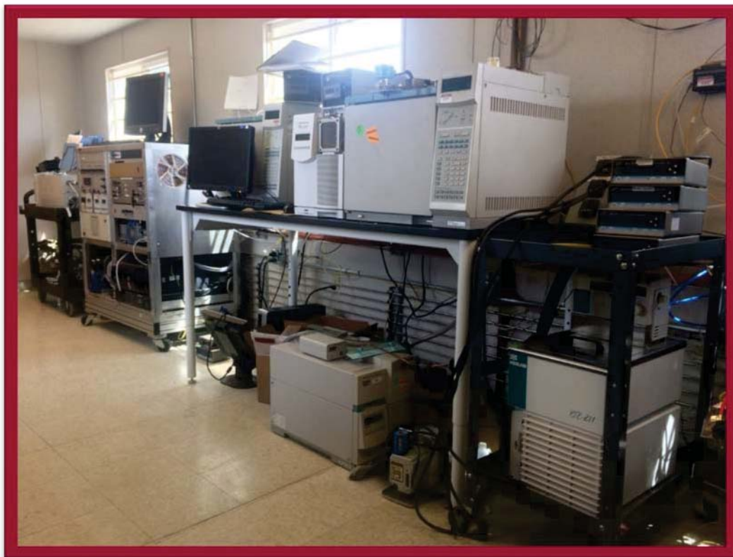
Figure 3. NUCON® Instrumentation Trailer
