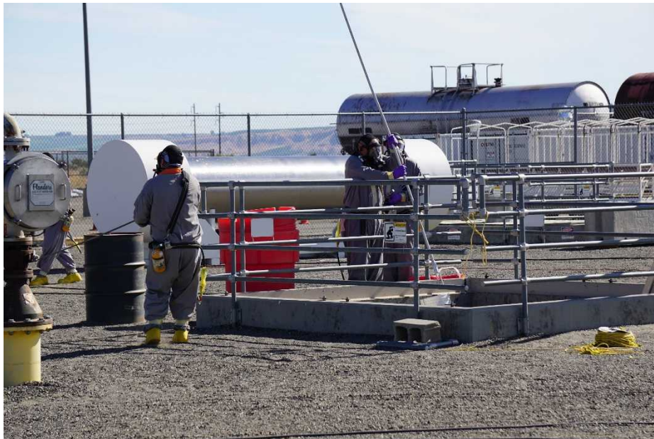
Figure 2. Mockup Demonstration at HAMMER – Using long-reach tools to remove equipment from a pit.
