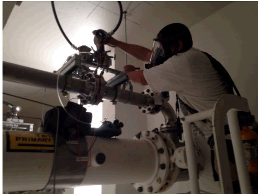
Figure 6. Field Trial in 241-AP Tank Farm - Performing AP Farm DST Flow Monitoring CAT in ventilation pit.
