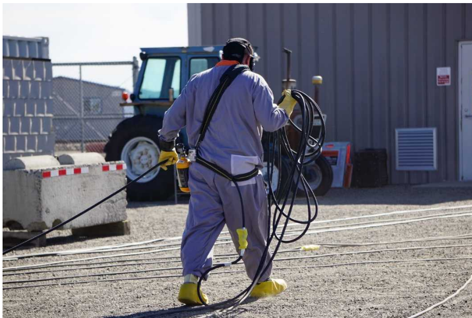
Figure 4. Mockup Demonstration at HAMMER – Carrying airline towards exit point.
