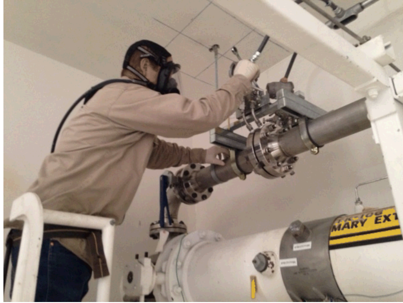
Figure 5. Field Trial in 241-AP Tank Farm Ventilation Pit - Performing AP Farm DST Flow Monitoring CAT .
