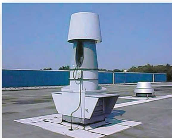
Strobic Air Dilution Exhaust System
