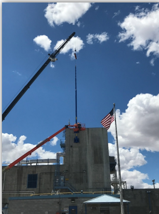
242-A Stack Installation – June 2017
