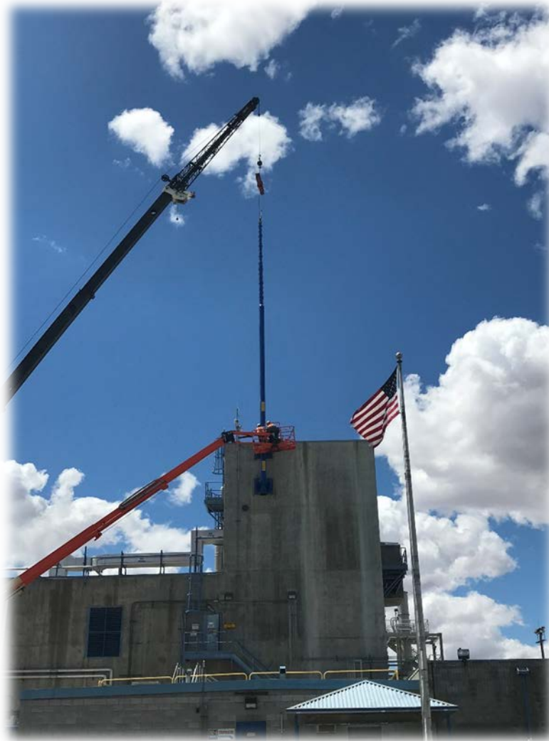
242-A Stack Installation – June 2017
