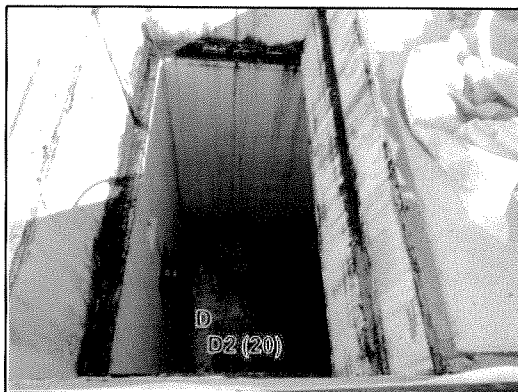
AY-02C Pit opened prior to temporary cover installation
