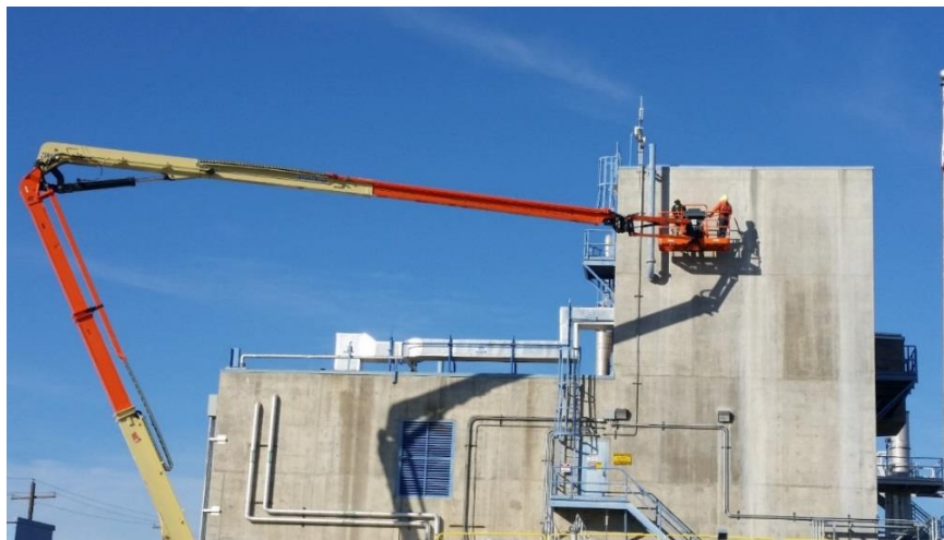
Figure 3. Construction Crew Completing the Facility Scans/Measurements on the 242-A Stack
