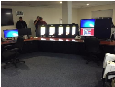
Figure 2. Construction Acceptance Testing TFSPS Annunciator in 274AW Central Control Room
