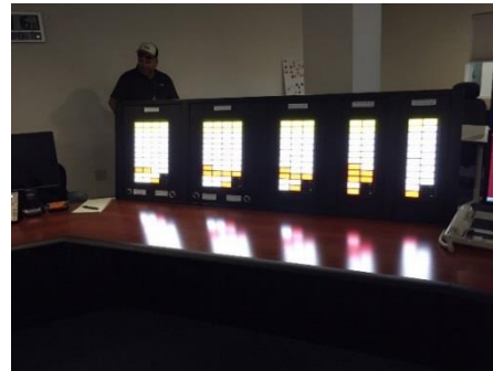
Figure 2. Construction Acceptance Testing TFSPS Annunciator in 274AW Central Control Room
